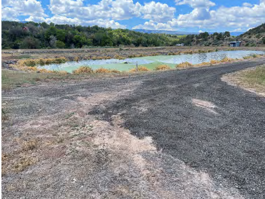
Figure 14. Access Road at the Headworks Building
