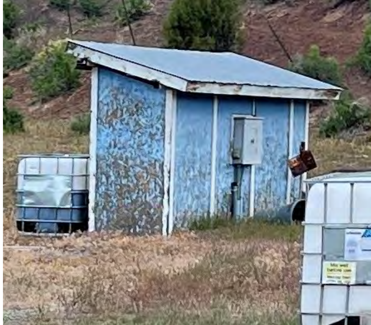
Figure 17. Influent/Headworks Building Exterior
