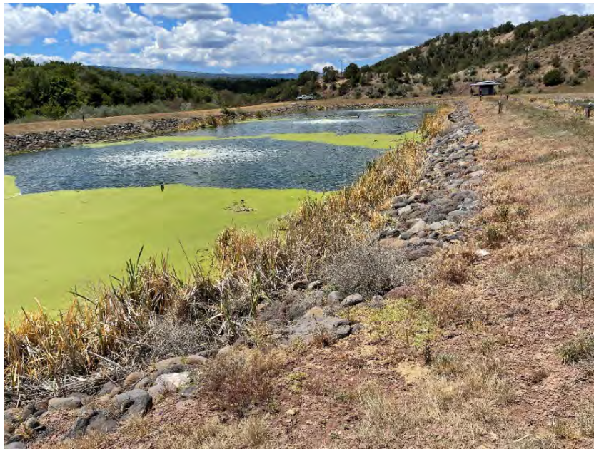
Figure 24. Cell No. 1 Berm Condition
