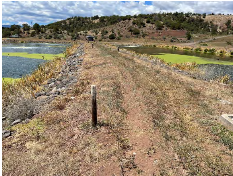
Figure 22. Cell No. 1 and Cell No. 2 Berm Condition
