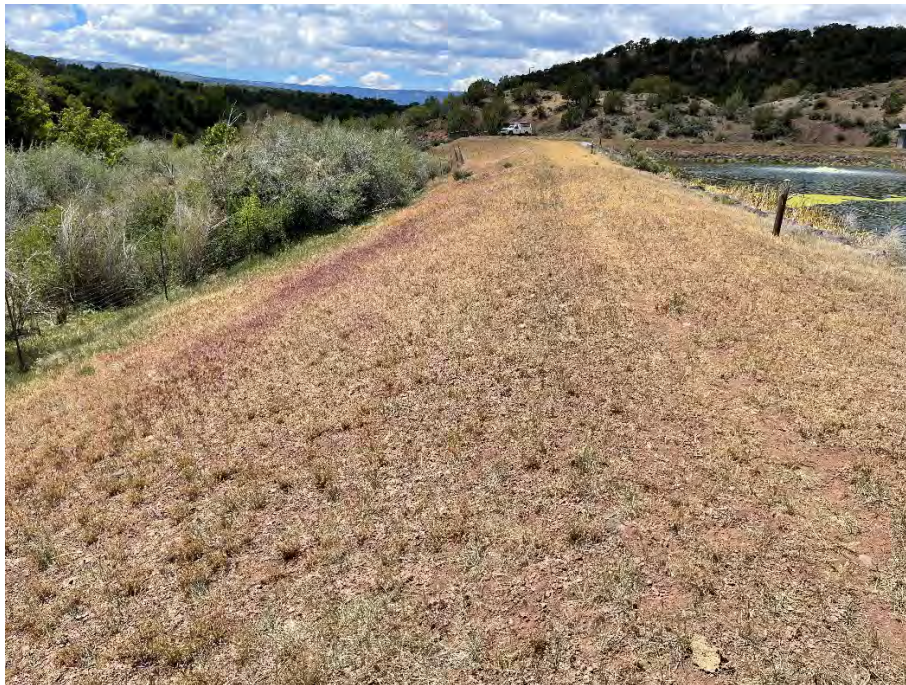
Figure 13. Access Road around Cell No. 1
