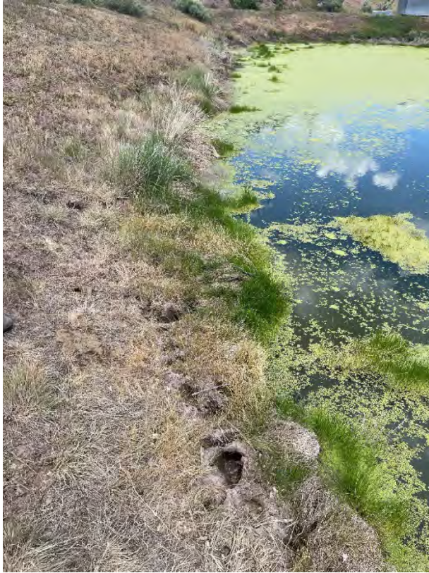
Figure 25. Settling Pond Berm Condition
