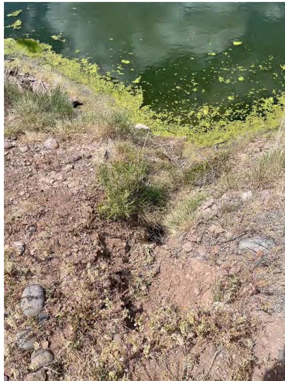
Figure 26. Settling Pond Berm Condition
