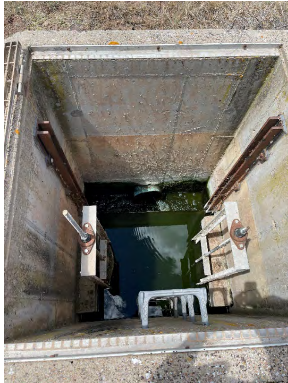
Figure 27. Cell No. 1 and Cell No. 2 transfer structure condition
