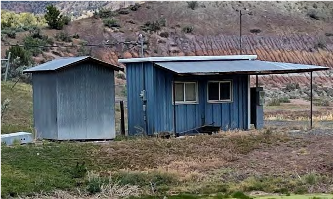
Figure 19. Control Building/Lab Exterior
