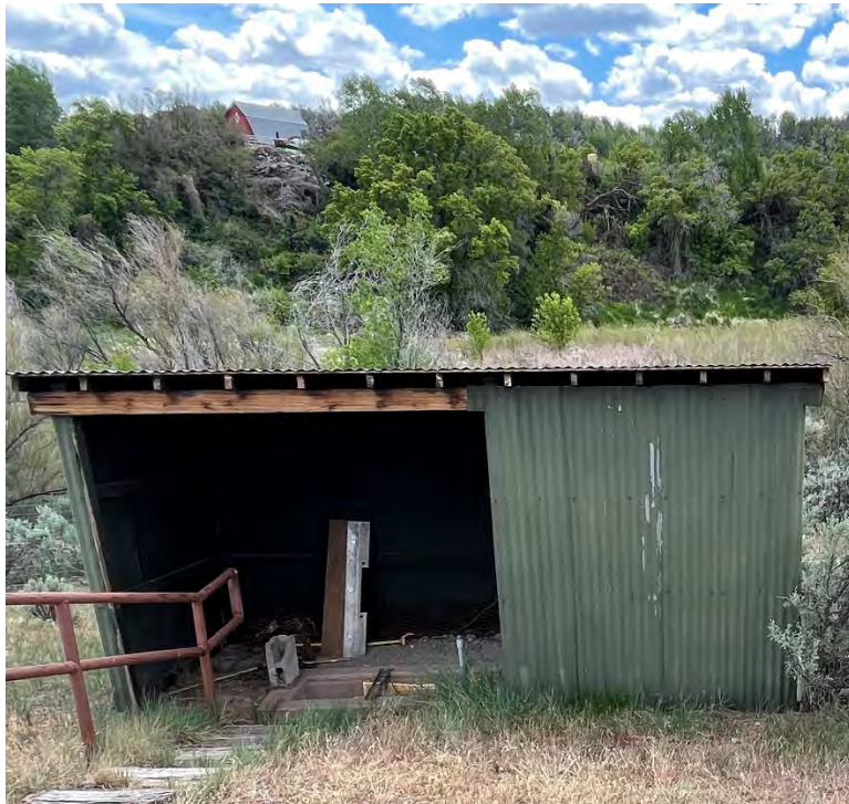
Figure 29. Chlorine structure condition
