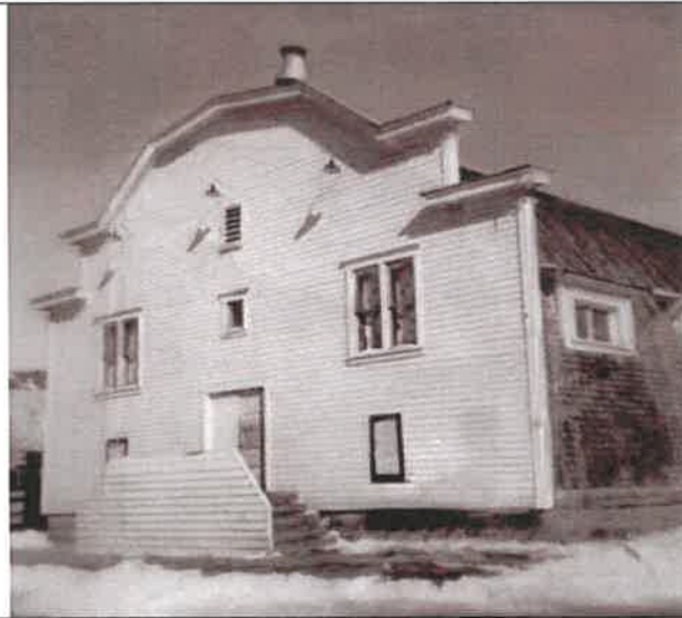
H5: Undated photo showing the addition of siding as a guardrail for the west entry stairs.
