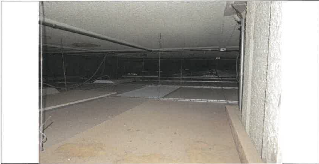
29: Space between the grid ceiling below and original ceiling above.
