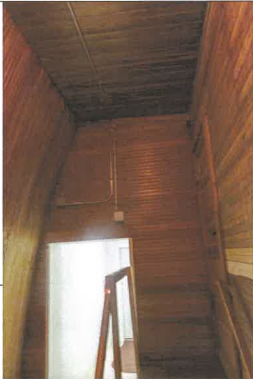
27: Hallway 105 east view with surface mounted electrical conduit and added stair handrail.
