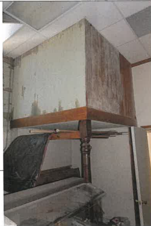
18: Storage 103 projection room column.
