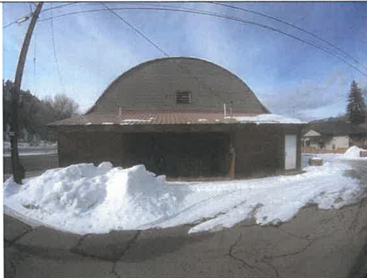
2: East Elevation: the shed roof and T-111 bump outs are not original, the basement is accessed in the east elevation below the shed roof and between the bump outs.
