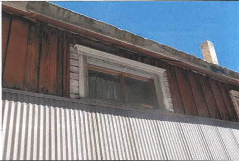
9: South Elevation clerestory window with original drop siding visible.
