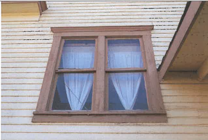
7: West façade – north double hung window set.
