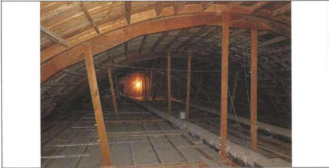
30: Attic bow truss roof framing with bowed 2x6 girts spanning between.
