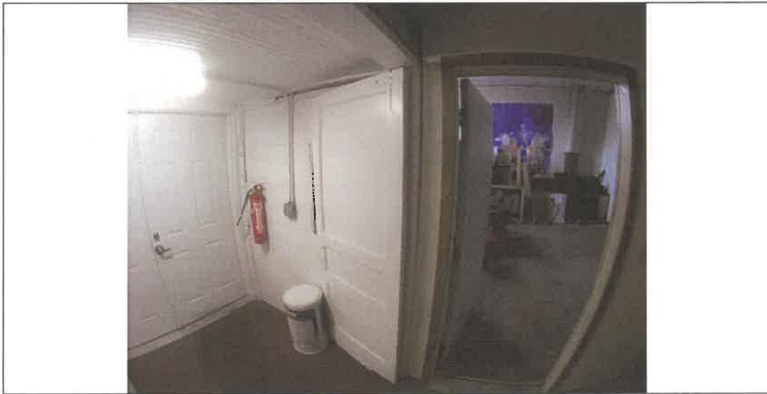
19: Entry Vestibule 101 with pivot doors.
