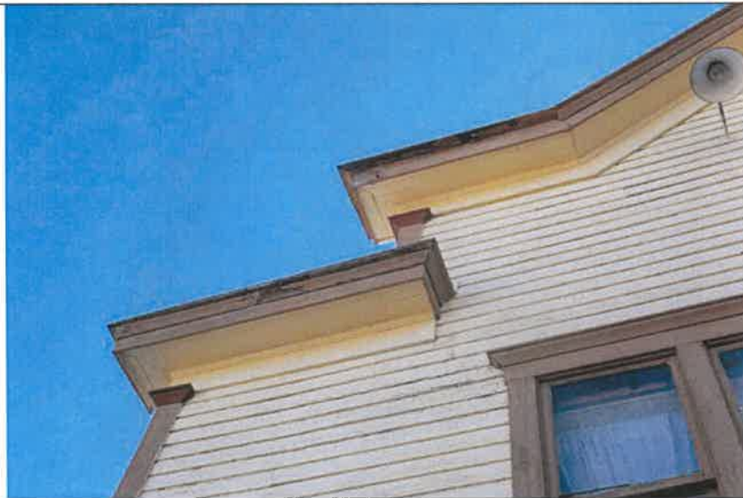
6: West façade – north cornice detail.
