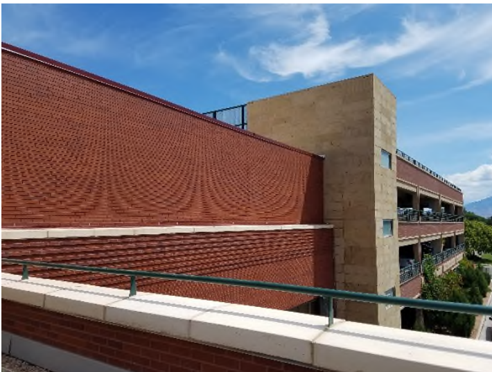
CMU University Center Expansion
