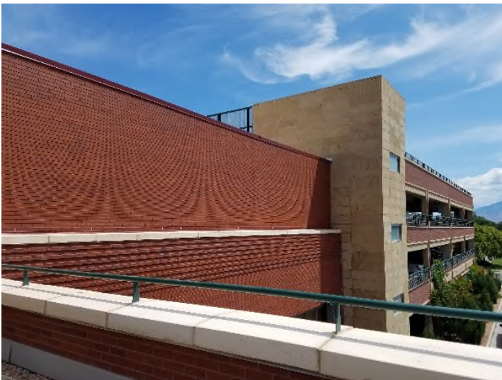
CMU University Center Expansion
